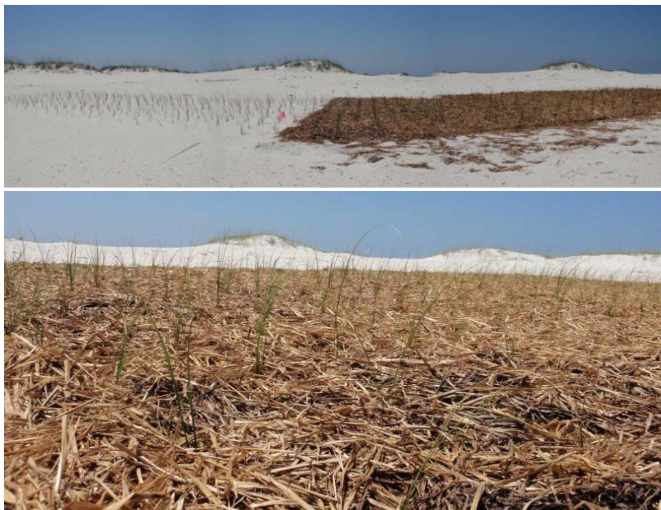
Figure 23. Foredune restoration site of sea oats ( Uniola paniculata ) planted approximately 12 in apart, the right half with an 8-inch layer of wheat straw two weeks after planting to serve as an artificial wrack. Below, the close-up view.
