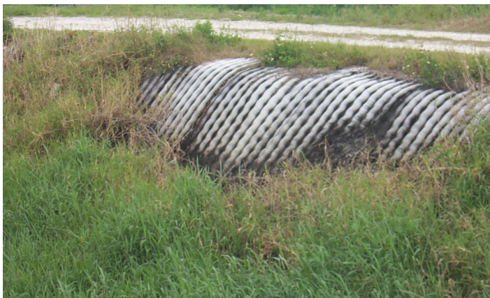
Figure 5. Canal bank stabilization in a high velocity area using a hardened synthetic ground covering. Credits: PCW
