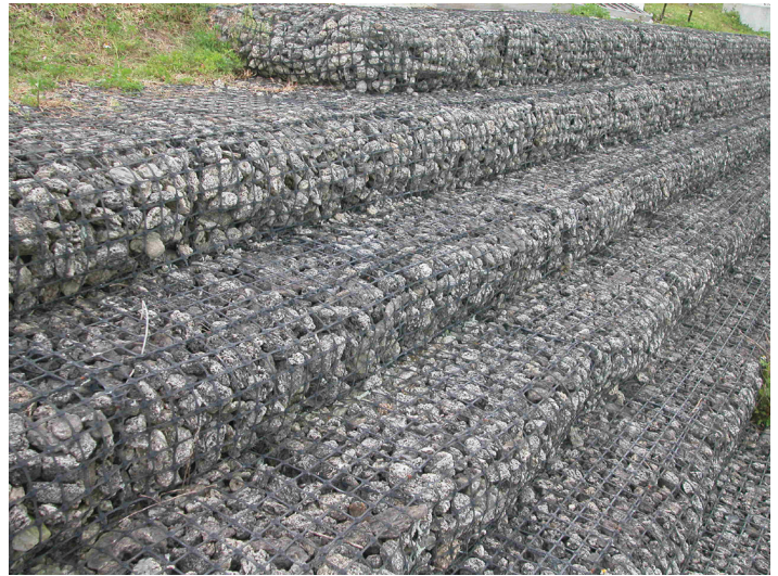
Figure 6. Use of gabions for stabilization of a canal side-bank. While expensive, these materials effectively prevent erosion in canal/ditch areas subject to high flow velocities.
