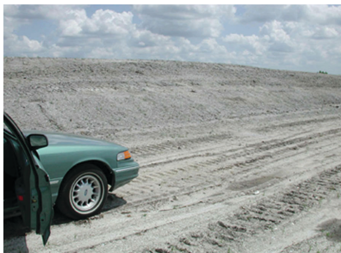
Figure 1. Coarse sediments removed from an agricultural canal. These sediments settled over several decades. Fine particle fractions likely deposited in the St. Lucie estuary, where water velocities are low. Credits: PCW
