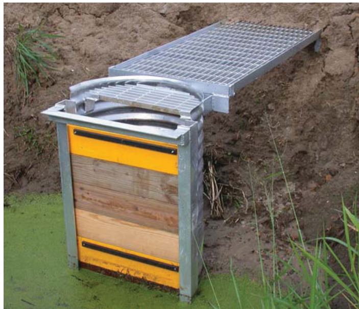
Figure 5c. Riser-board structure with two sinker boards installed. The sinker boards should be brightly colored to facilitate retrieval if they are accidentally dropped in the ditch or misplaced around the structure. Credits: PCW
