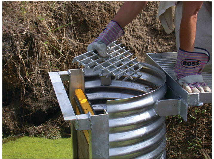
Figure 7a. Removable foot support plate on top of structure. When used, support structures should be routinely inspected and repaired if cracks, corrosion, or other signs of weakness are observed. Credits: PCW
