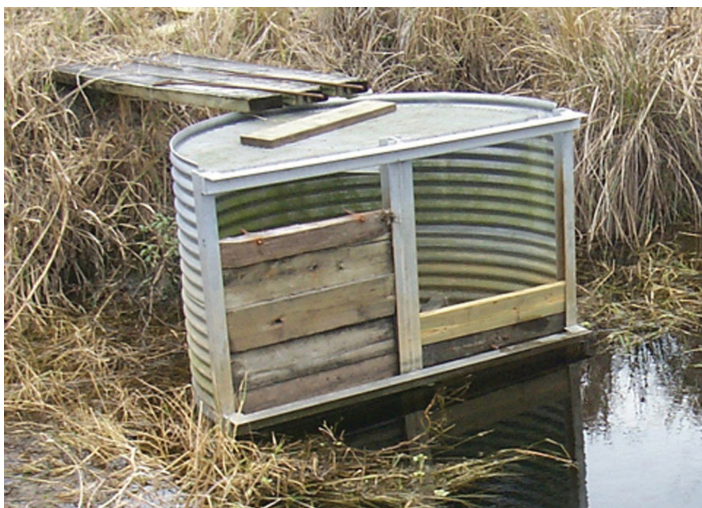
Figure 2. Typical riser-board structure within a citrus grove drainage system. Note: Wooden catwalks should be routinely inspected for decay. Wood degrades relatively quickly in the environment, exposing operators to increased dangers associated with breakage or slickness. These catwalks should also be wide enough to allow easy access for workers, without requiring a balancing act. Credits: PCW
