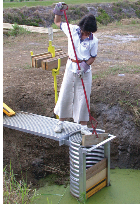
Figure 3. Tools needed for safe operation of a riser-board structure include gloves and long-handled tools (such as modified ice tongs) for removing/inserting boards. Always wear gloves when working around riser-board structures.
