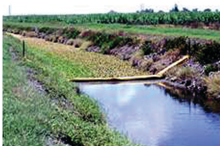
Figure 11. Weed booms (a) and trash racks (b) keep aquatic weeds from drainage pumps.
