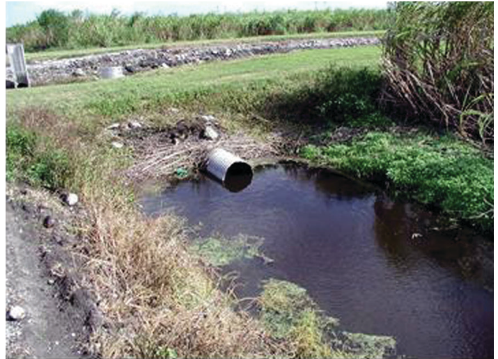
Figure 9. Raised culvert bottom reduces bedload sediment transport.
