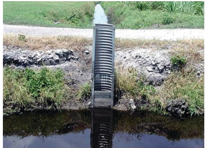
Figure 7. Riser boards slow drainage near pumps.
