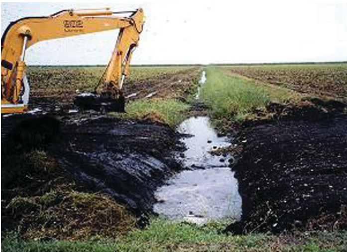
Figure 6. Removal of soil and sediment buildup in field ditches.
