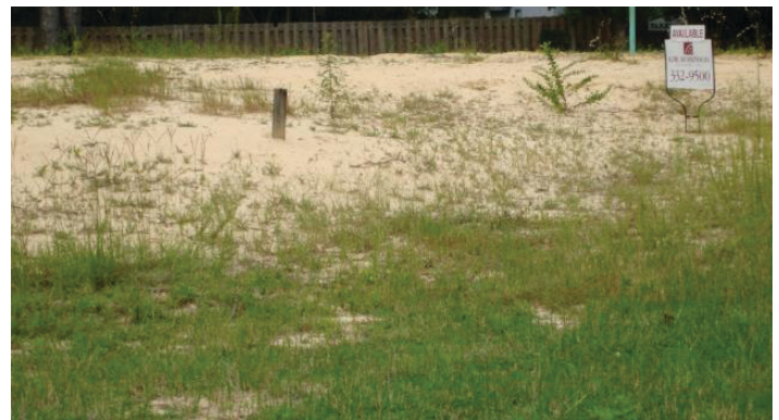
Figure 1. Fill sand is often piled on construction sites to serve as a base for the home's foundation. Credits: George Hochmuth
