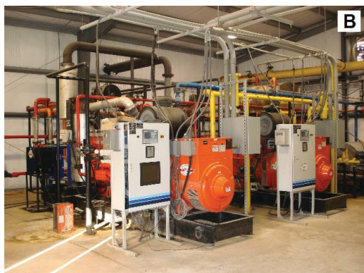
Figure 9. The biogas is transported to the CHP systems through transportation pipes (A) to the engine/generator room (B) where it is burned to turn a generator.
