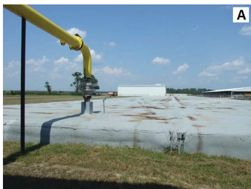
Figure 8. (A) Manure and bedding mixture is being loaded into (B) the mixed plug-flow anaerobic digester (biogas is unloaded at the far end).
