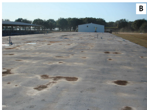
Figure 8. (A) Manure and bedding mixture is being loaded into (B) the mixed plug-flow anaerobic digester (biogas is unloaded at the far end).
