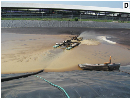
Figure 10. Storage systems for (A) digested solids and (B) liquid effluents generated from anaerobic digestion of beef cattle manure. The round tank (C) further separates solids from the liquid fraction where heavier fractions settle out and the liquid flows to the storage pond where the effluent is filtered (D) before being injected into the irrigation system for field application.
