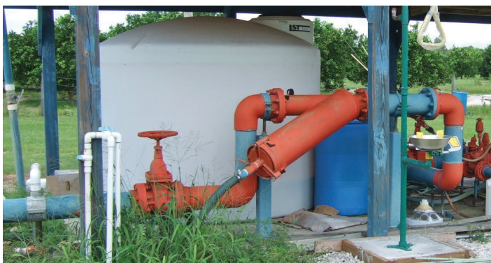
Figure 2. Nutrient solution sources for fertigation are stored in large plastic tanks at the irrigation pump station.
