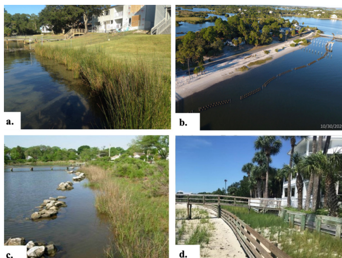
Figure 1. Examples of living shorelines. Living shorelines can take many forms. For example, they may include shoreline buffers made of only vegetation as in panel a, or they can include elements such as sills of materials made to recruit oysters (panel b) or rock breakwaters (panel c). The living shoreline in panel d includes two zones of vegetation (high and low marsh, separated by a fence) deployed adjacent to a bulkhead structure.
