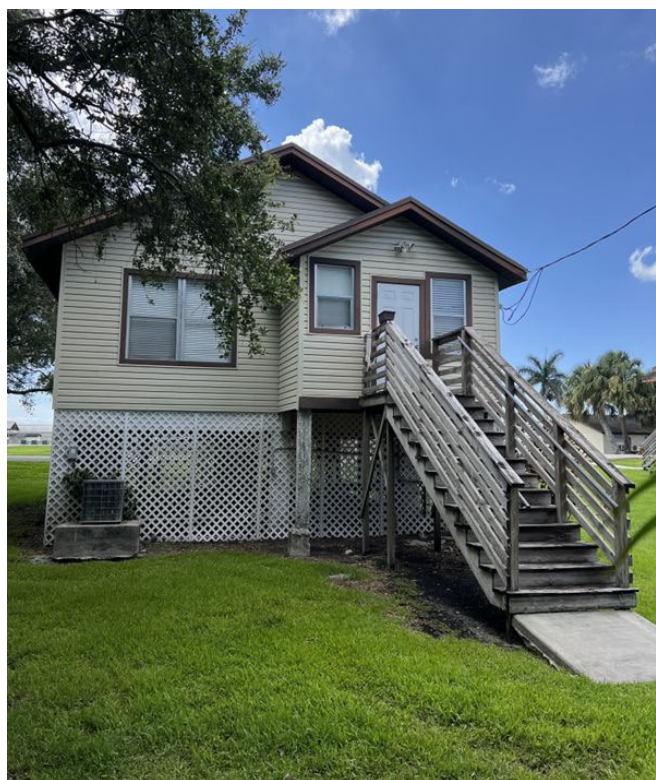
Figure 1. This building, located at the UF/IFAS Everglades Research and Education Center, was originally constructed at ground level in the 1920s. Through time, significant organic soil loss necessitated the addition of latticework and stairs to support the structure.
