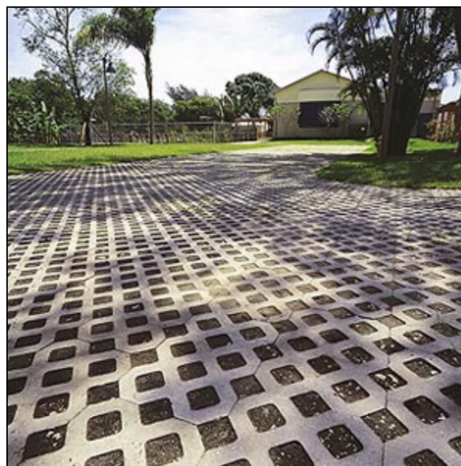
Figure 1. Pervious pavers are designed to promote vehicular and pedestrian traffic in land areas that would otherwise be unusable due to stormwater retention. Impervious pavement systems, such as asphalt, promote heat and stormwater runoff. Pervious pavers provide a natural way to let water percolate to the ground, while still offering a durable and aesthetically pleasing pavement surface.
