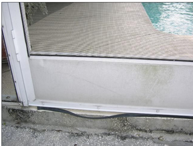
Figure 3. Door sweeps can prevent snakes from inadvertently slipping into the home under a door, butdoor butchecked periodically. This rubber door strip is in disrepair, leaving large gaps beneath the door.
