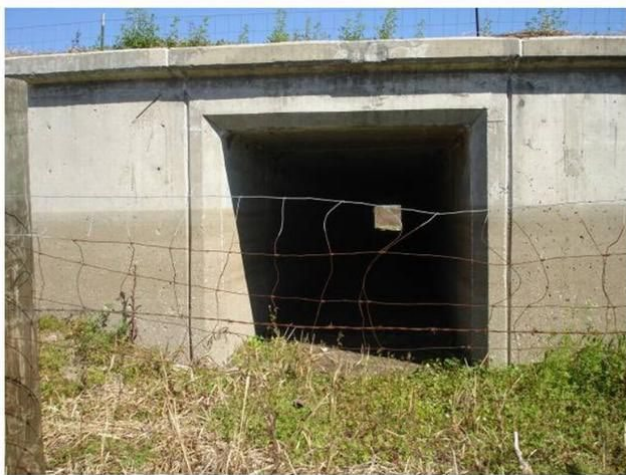
Figure 1. A wildlife box culvert under a four-lane road that passes through Paynes Prairie State Park, Florida. A number of reptiles, amphibians, and mammals use this wildlife passage. Credit: Dan Pennington, 1000 Friends of Florida
