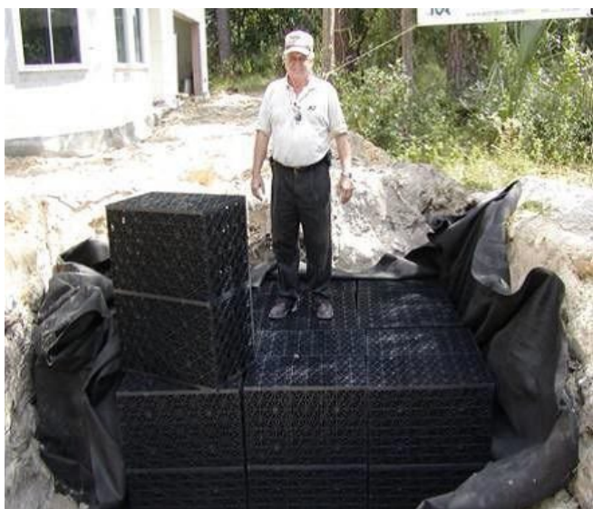
Figure 4. A subsurface exfiltration system installed at the Madera subdivision in Gainesville, FL. Program for Resource Efficient Communities, University of Florida 2004
