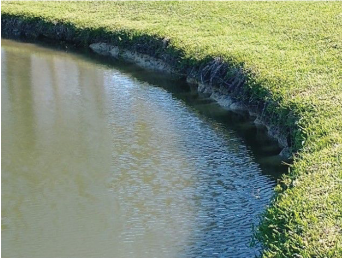
Figure 2. Erosion can result in a steep, unsafe pond bank. Credits: Michelle Atkinson, 2021, UF/IFAS
