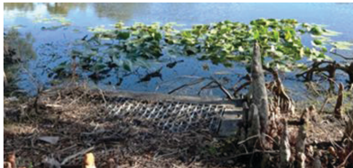
Figure 9. Drainage structures need to be kept clear of debris. Credits: Michelle Atkinson, 2022, UF/IFAS
