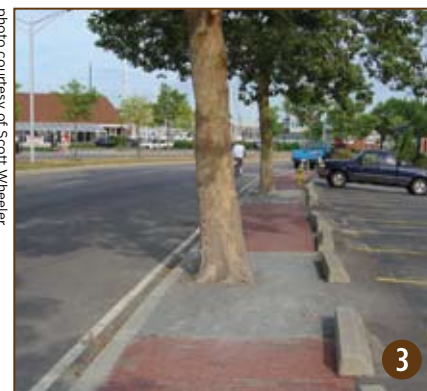
Figure 3 Stone dust is placed around the root flare of the tree in cutouts along this brick sidewalk. This technique is attractive and allows for easy repair as roots expand in diameter.
