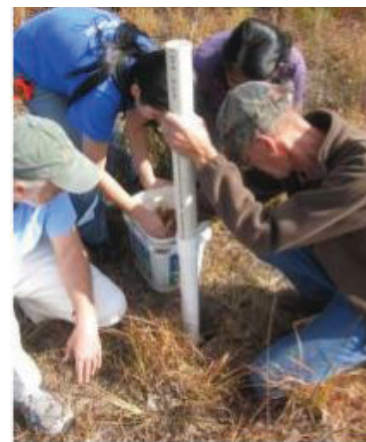
Figure 1. Citizen scientist volunteers assist in the installation of groundwater monitoring wells.
