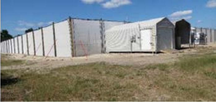
Figure 4. The UF/IFAS CREC CUPS facility near Lake Alfred, FL. Credits: Arnold W. Schumann, UF/IFAS
